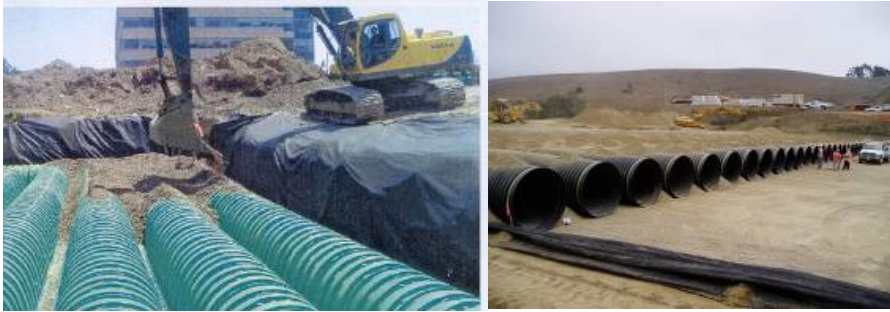
Figure- Triton S-29 Chambers with EPDM liner
