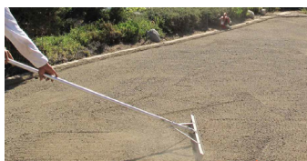
3 Spreading the Base
