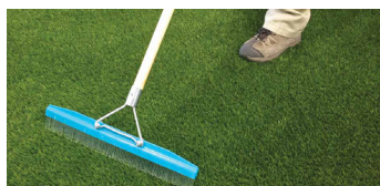
9 Spreading the Infill
